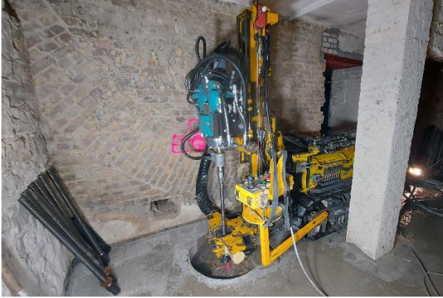
(1) A KLEMM KR 701 was used for the anchor drilling work.
