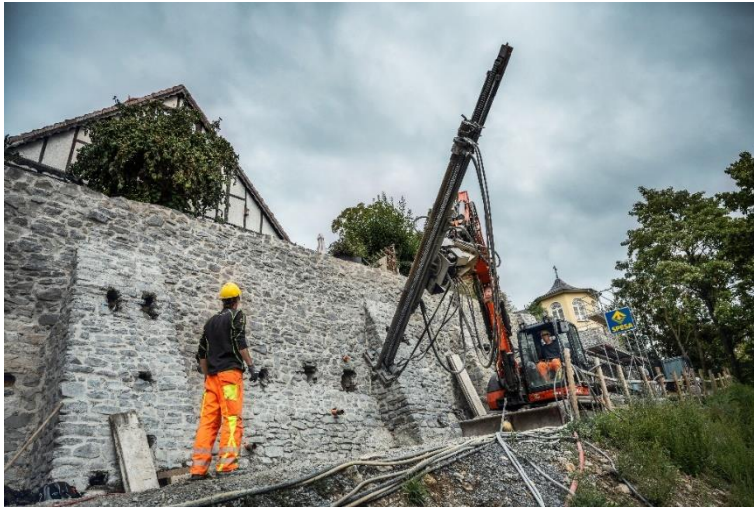
(3) Injection boreholes and masonry nails were installed along with structural reinforcement using self-drilling anchors.
