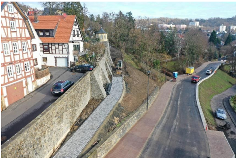
(4) Nearly completed project shortly before opening for traffic
