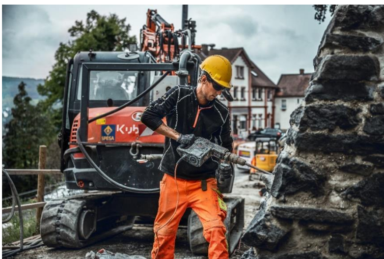
(2) One of the most laborious tasks involved chiseling out the existing damaged wall joints over an area of 400 m 2 .
